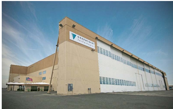
Greenpoint’s hangar facility in Moses Lake, Washington
